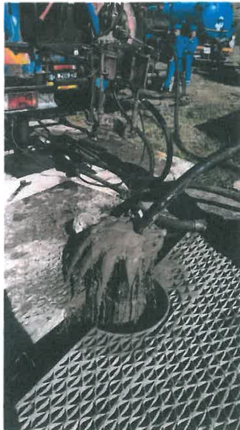
Coloana 8 5/8 in umpluta cu ciment
