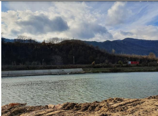
Aval nod hidrotehnic – dig mal drept partial realizat
