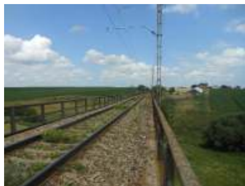
Viaduct km existent 20+660
